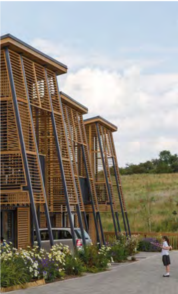
At Hanham Hall SIPs panels were used to accelerate delivery, enhance performance and create the overhang for the entrance veranda
