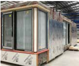
Modules under construction in the factory
