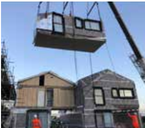
Modules being delivered to site
